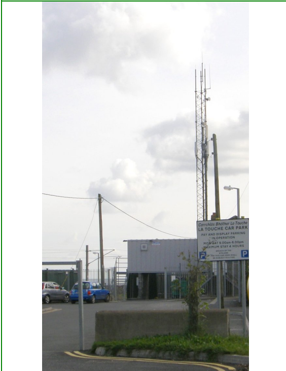
Transmitter Site Photo
